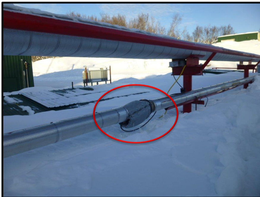
December 30, 2013 - Installed HydroFLOW 120i with winter protection (0° F / -18° C)
