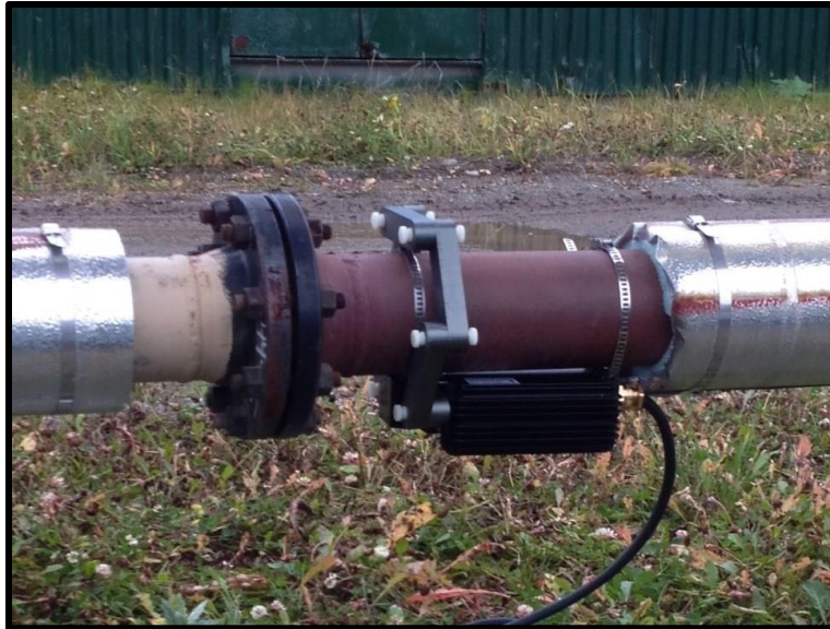
December 30, 2013 - Installed HydroFLOW 120i with winter protection (0° F / -18° C)
