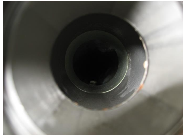
Treated E1 nozzle – 30' down the line
