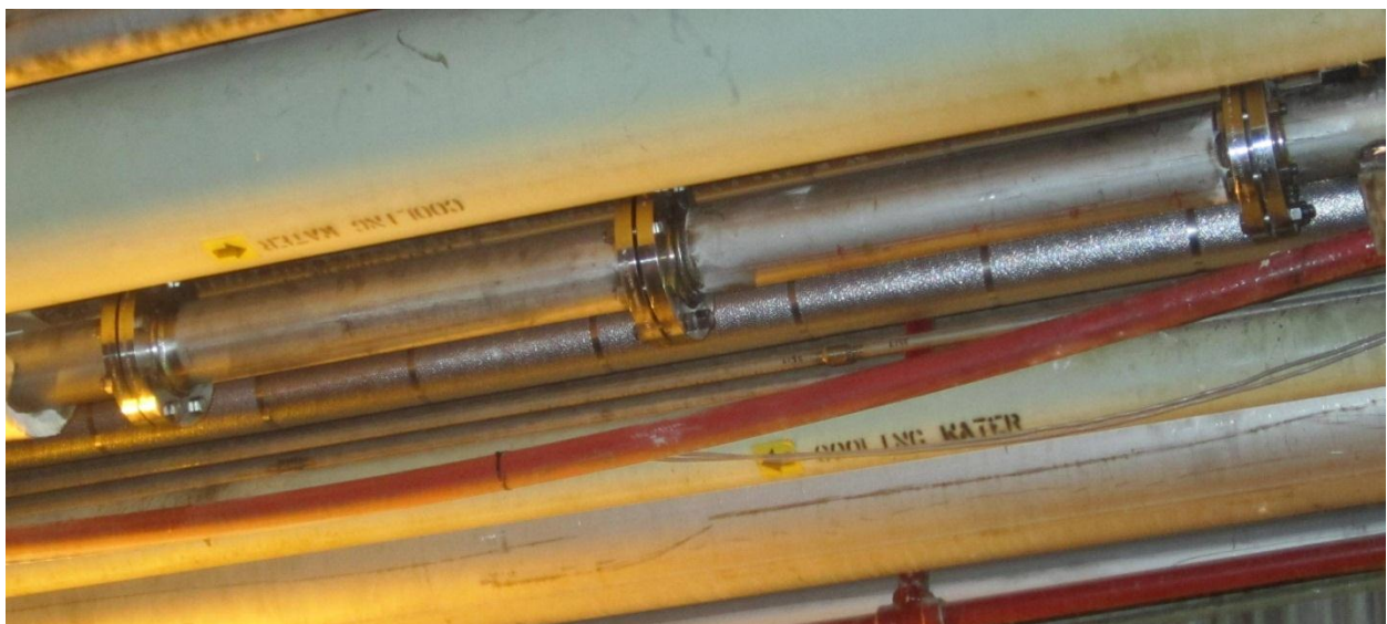
Contaminated and clean 30" [762mm] pipe spool sections
