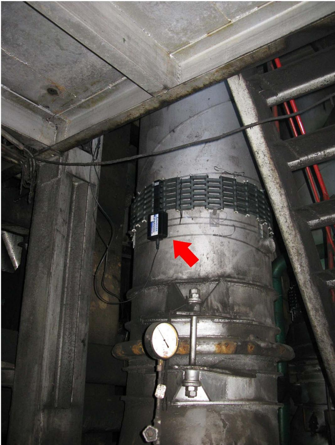
AquaKlear Custom P-40” is installed on a pipeline.
