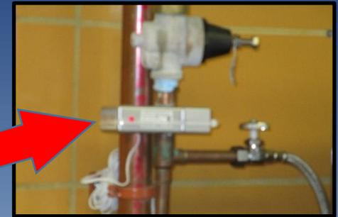
*HydroFLOW* S38 installed on cold water supply line feeding the steamer oven
