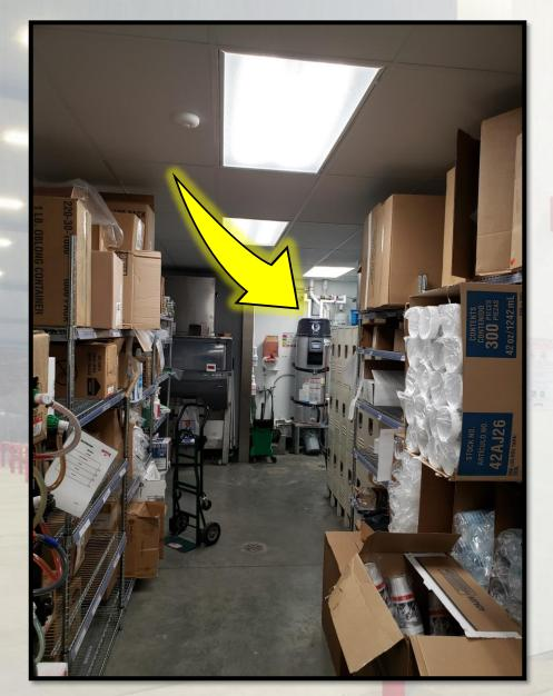
**Newer stores** have a 1 1/4 inch cold water pipe entering the water heater. **These stores** require an hs40 device.
