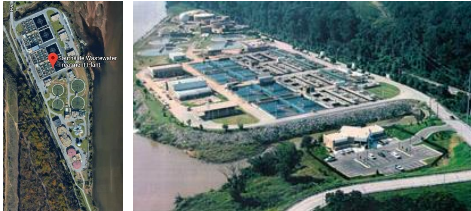
Figure 2. The Southside Wastewater Treatment Plant
