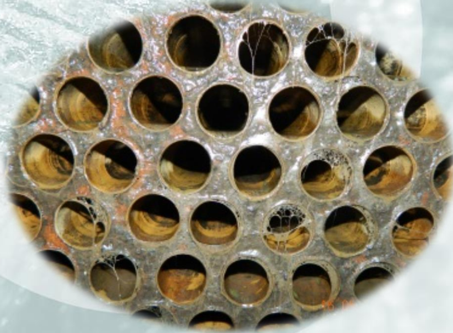
After the custom 56" units was installed - Tubes free of biofilm
