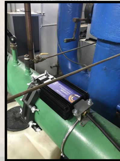
Installed HydroFLOW devices
