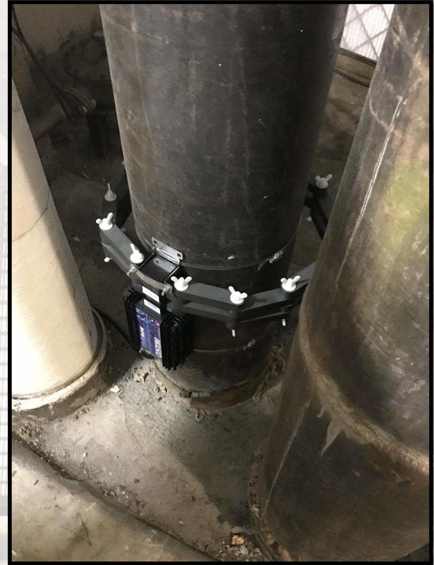
Installed HydroFLOW i14" device
