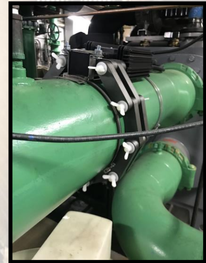
Installed HydroFLOW devices
